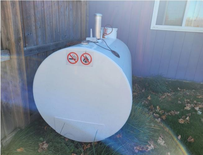
PHOTO 19: Close up of Fuel AST observed at north adjacent to the building at 513047 2nd Line, Amaranth.
