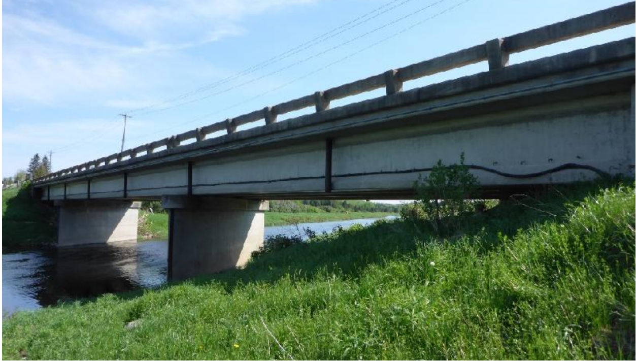
(S1) Structure 004-0142 Bridge No. 1 – West Elevation
