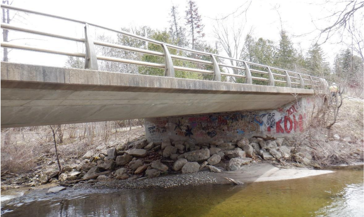
(S3) Structure 030-0318 Nottawasaga Bridge – Pre-Construction North Elevation
