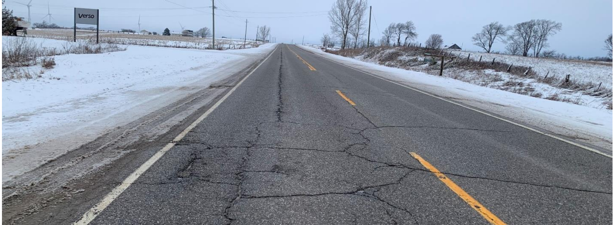
(R1) Dufferin County Road 124 – Pre-Construction Photo
