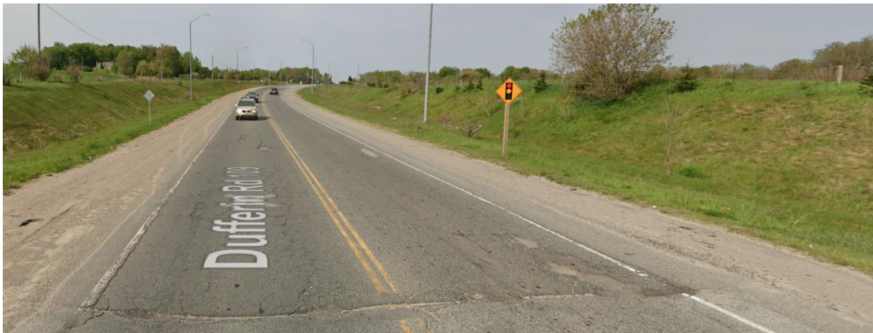
(R2) Dufferin County Road 109 South Arterial Road – Pre-Construction Photo
