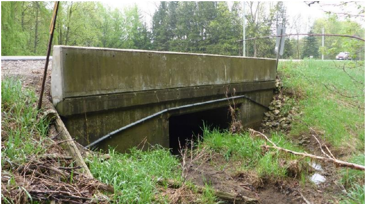
(S2) Structure 004-0901 Culvert 501 – West Elevation
