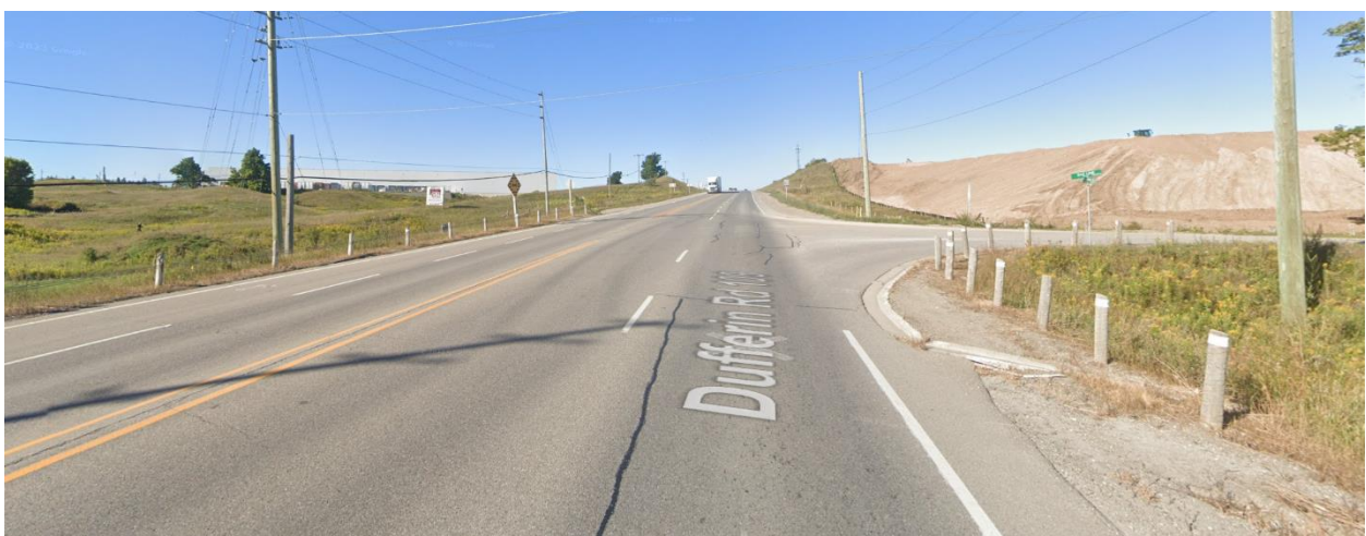
(R3) Dufferin County Road 109 at 2 nd Line Intersection – Pre-Construction Photo
