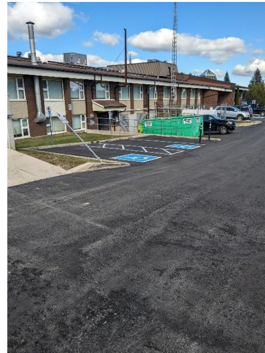
Mel Lloyd Centre parking lot, Entrance E, Accessibility spots
