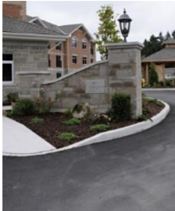
Lawrence Avenue Asphalt Paving
