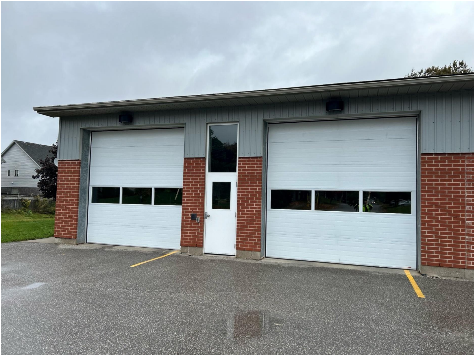
Shelburne Paramedic Building Garage Doors
