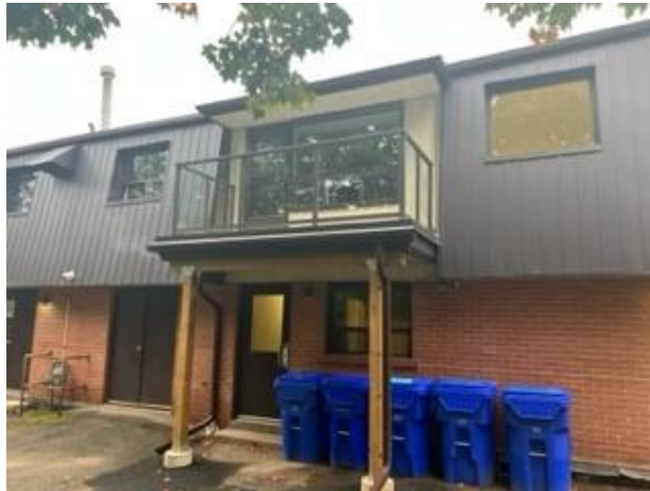
William Street Balcony Replacement
