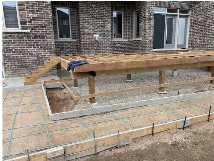
Deck Building Inspection
