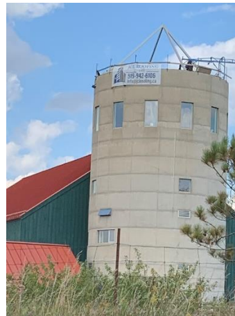
Museum Silo Roof Replacement
