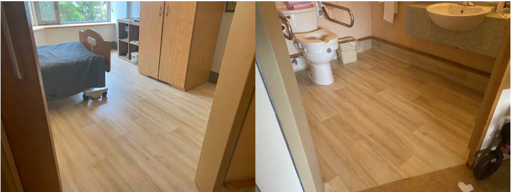
Resident room flooring upgrades
